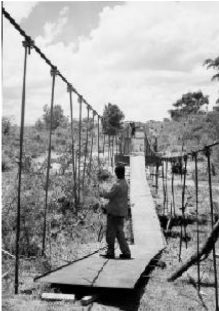
Lifting of the deck platform using chains and tensioners during the construction of the Murerezi suspension footbridge, Zaka Rural District Council, Zimbabwe
