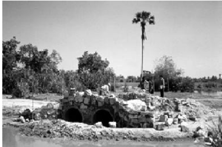
Culvert construction, Svay Rieng Province, Cambodia
