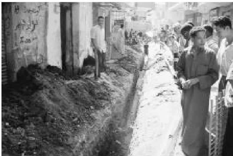
Rehabilitation of a water supply network in Cairo Governorate
