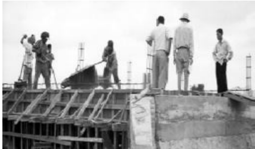
Bridge works, Kandal Province, Cambodia
