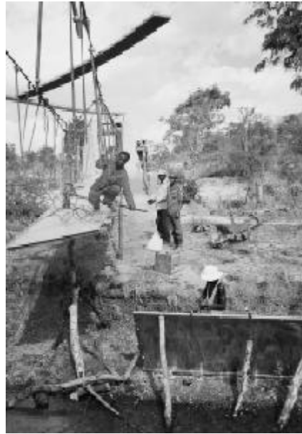
Lifting of the deck platform using chains and tensioners during the construction of the Murerezi suspension footbridge, Zaka Rural District Council, Zimbabwe
