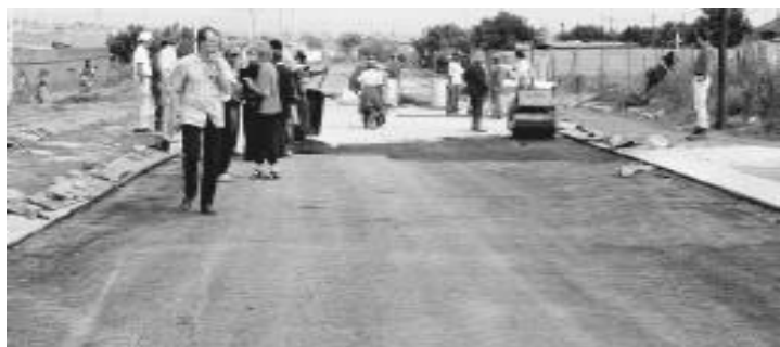
Emerging contractors surfacing a road using labour-based techniques
