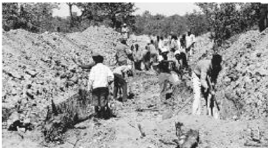
Excavating for wearing course material in Namibia
