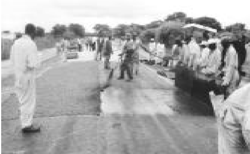
Labour-based road surfacing trials in Inkosikazi, Zimbabwe
